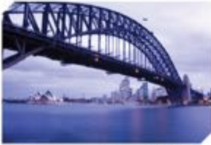
Sydney Harbor Bridge, Australia
