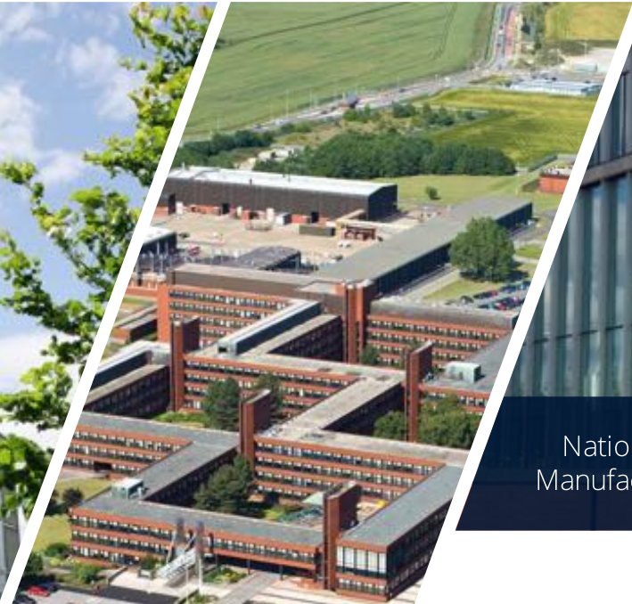
National Industrial Biotechnology Facility
